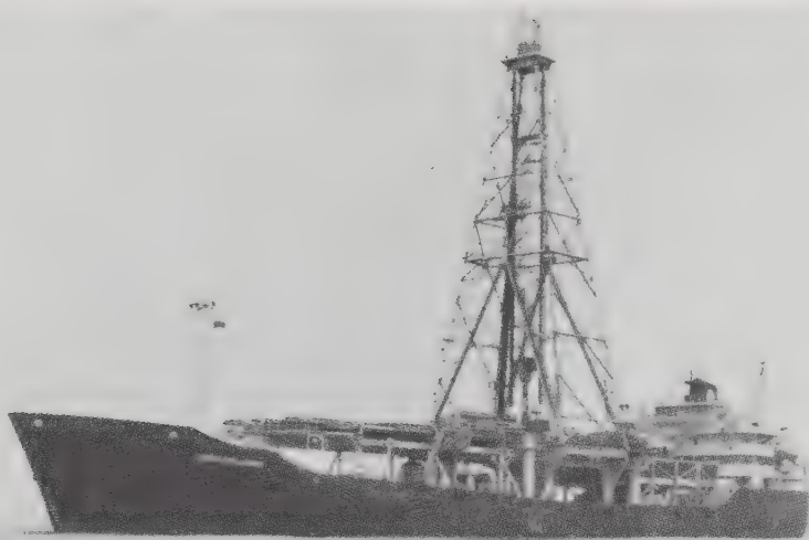
Fig. 1.13. Deep-sea drilling vessel Glomar Challenger . Since 1968, owned by Global Marine Inc., Los Angeles, operated by the Scripps Institution of Oceanography, La Jolla, Calif. for JOIDES. Length 131 m, displacement 10,500 tonnes, height of the drilling tower 59 m above the water line, operating at water depth down to 6000 m, penetrates into the sea floor as far as 750 m. Photograph courtesy of Scripps Institution of Oceanography.
