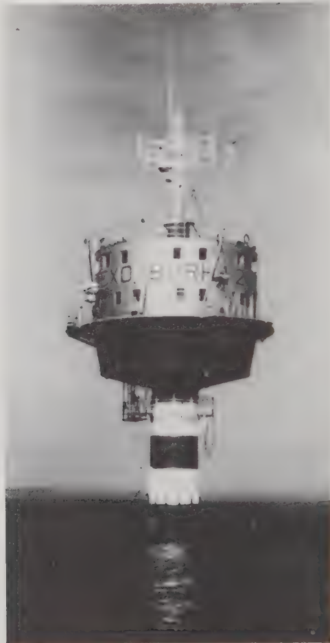
Fig. 3.11. Moorable manned surface buoy Borha II . Total height 79.3 m, 60 m of which are immersed. The diameter at the head of the buoy is 10 m, at the sea surface 2.8 m, at the foot of the buoy 7 m. The displacement is approximately 910 tonnes. Natural period: pitching motion 24 sec, rolling motion 28 sec (Photo: CNEXO, Paris).
